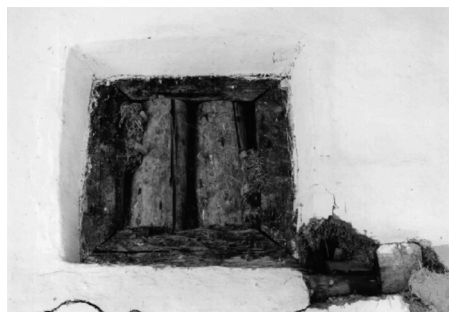
Figure 6. Čistá u Litomyšle , distr. Svitavy , farmhouse No. 171: detail of the smoke window of the living (all purpose) room. (Credits: Jiří Škabrada).
