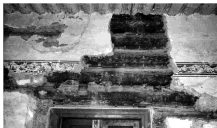
Figure 3. Vračovice, distr. Ústí nad Orlicí, farmhouse No. 2: secondary interior earthen coating of the former smoky room dated 1538 supported by wooden nails. (Credits: Jiří Škabrada).
