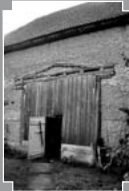
Fig. 10 : A barn door covered with a wooden strutted frame (C. Ziegert).
