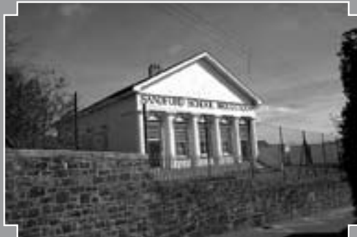
Fig. 2 : A cob building : the school in Sandford-1825 (L. Watson).
