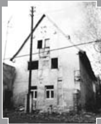
Fig. 4 : Cob building with timber-framed upper floor, Saxony-Anhalt, 1658 (C. Ziegert).
