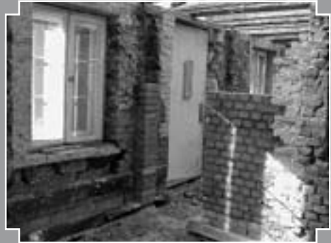
Fig. 16 : Installing horizontal moisture protection and replacing the damaged material with earth blocks during the reconstruction of a cob building damaged by dampness. Steinstücken near Berlin (C. Ziegert).
