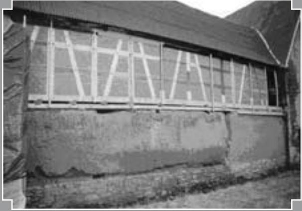
Fig. 15 : Cob wall damaged by rising dampness (C. Ziegert).
