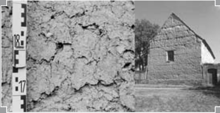
Fig. 12 : Example of a non-rendered wall showing a very slow weathering (C. Ziegert).
