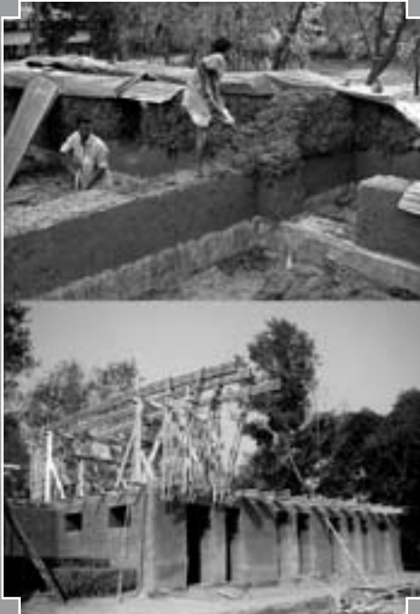
Fig. 18 : Stacking up of mud and bamboo beams supporting ceiling and upper floor (C. Ziegert).
